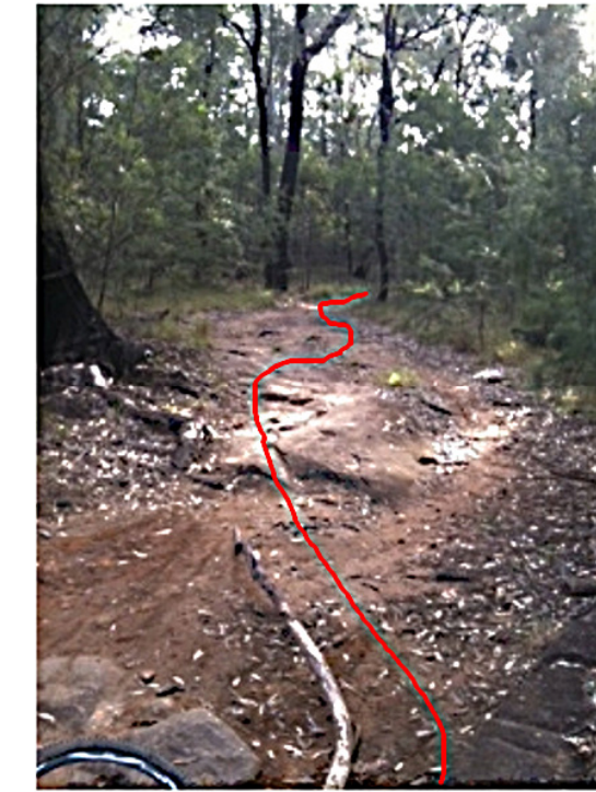
Looking up at the bottom. Large existing rock provides braking protection after final rock berm hip jump.
